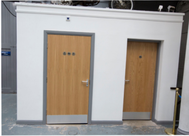
The ground floor toilets are in the transport gallery.
